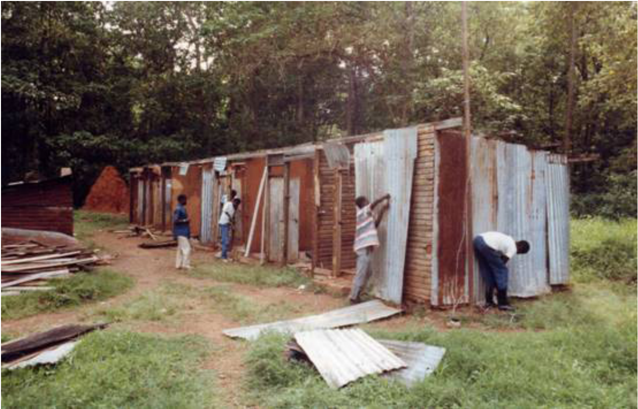
Old houses before renovation
