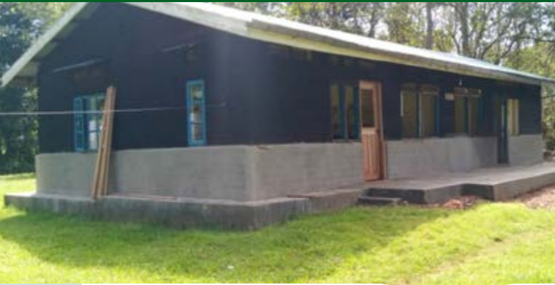
The basement of some houses were replaced with brick and concrete to provide a firm and safe base, but also aiming at minimizing the risk of termite infestation)
