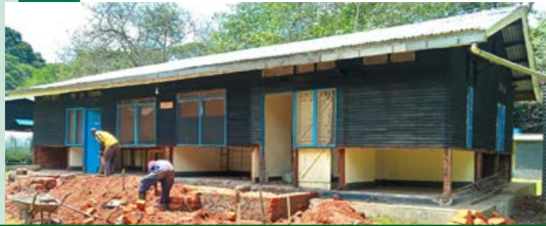
The basement of some houses were replaced with brick and concrete to provide a firm and safe base, but also aiming at minimizing the risk of termite infestation)
